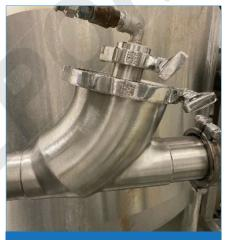
Figure 3. Ball Check Valve 1
