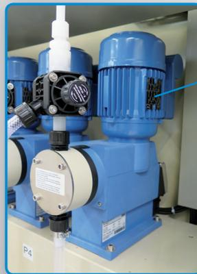
Elados diaphragm pumps with overpressure safety valves and/or snubbers against pressure shocks
